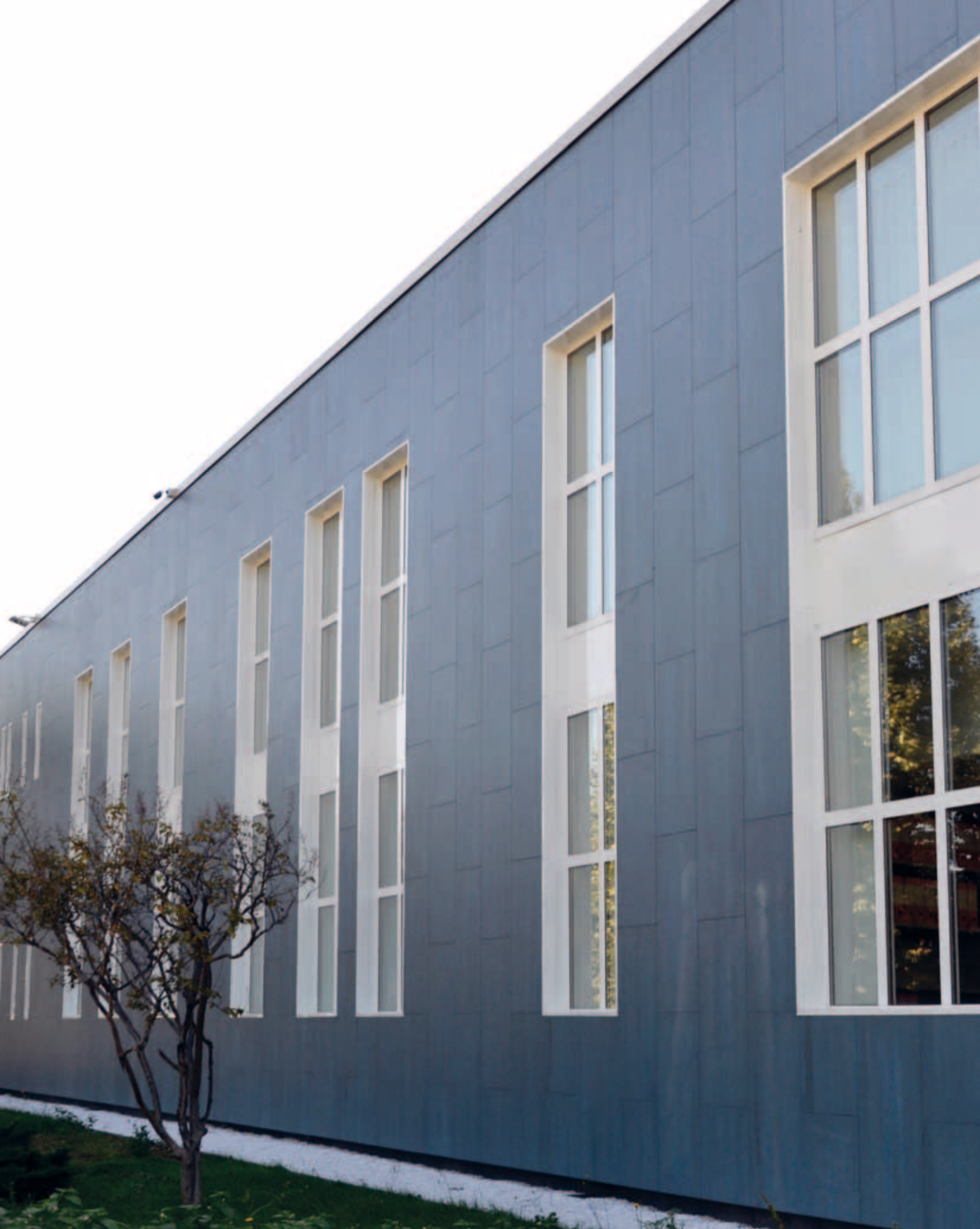
Evapco Europe Rho, Italia Alessandro Romeo, Cristiano Pizzi Marte: Azul Bahia cm 60x120
